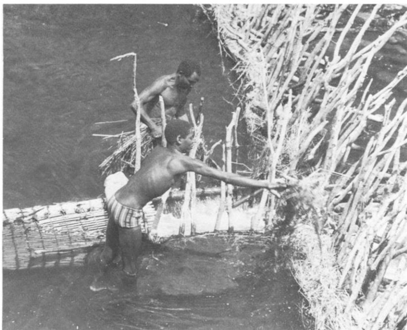
Replacing 'ndjagali' trap in fishing dam across Lufuko River near Lubanda. Man in background is stuffing straw into dam. A. Roberts, 1975.
